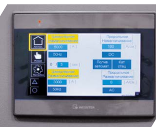
Sensor screen of power cabinet
